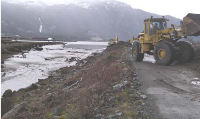
Construction begins March 7
