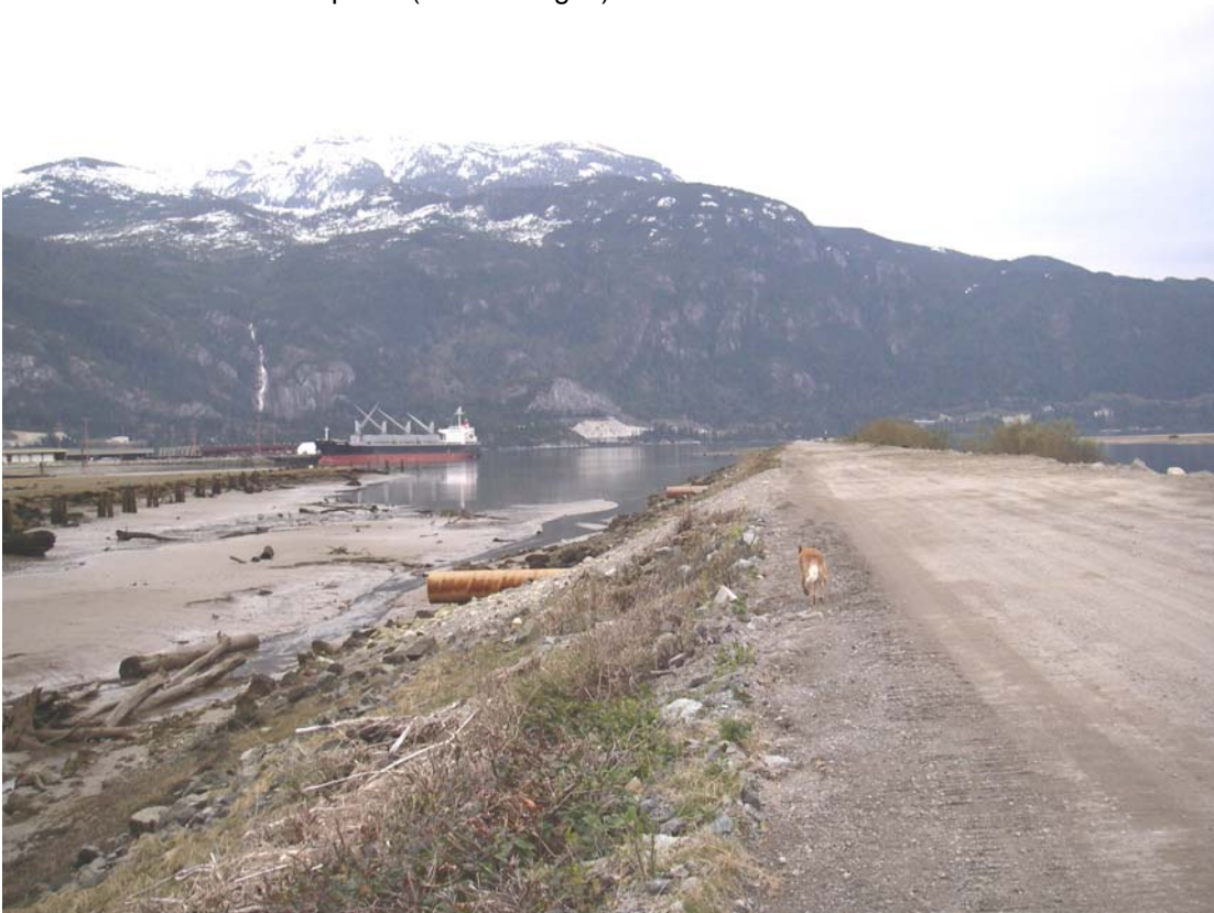
Second Culvert in place (low tide)
