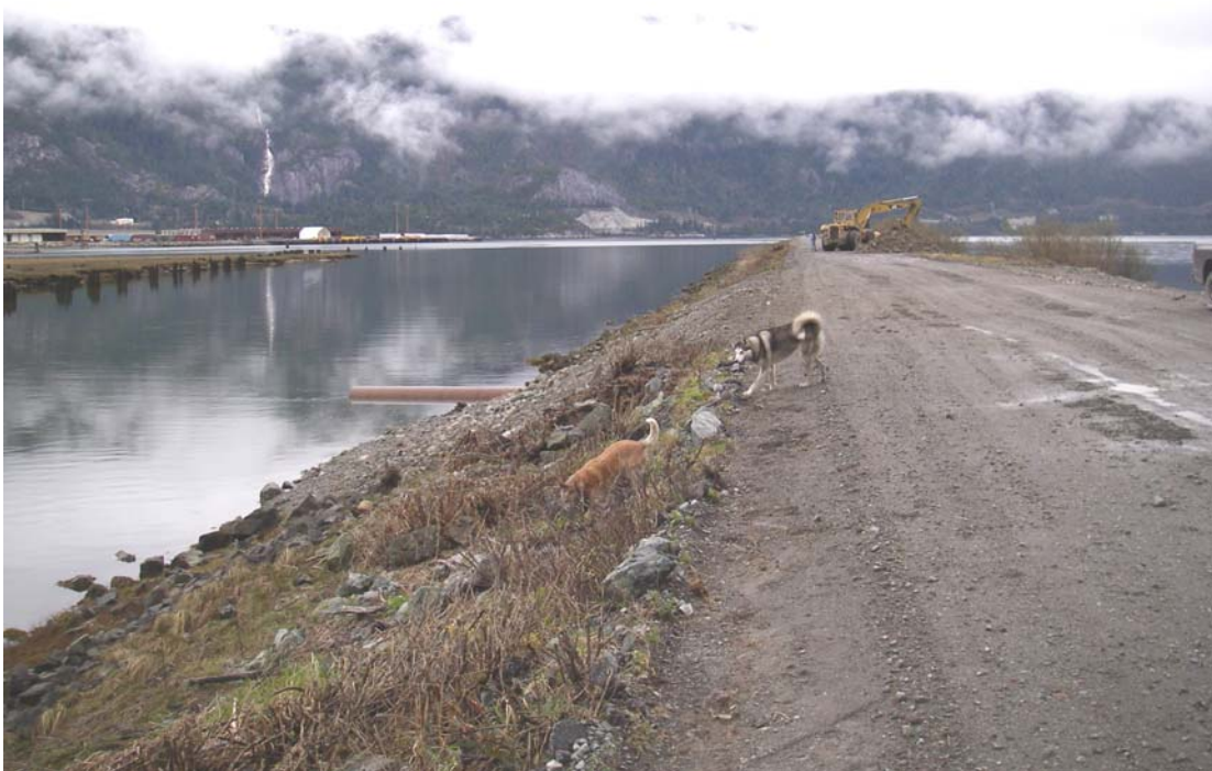
First Culvert in place (tide coming in)
