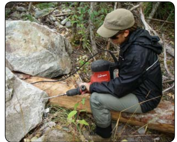
Creating boulder anchors for woody debris structure
