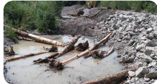
Mile 49 Channel - Completed LWD installation at the upstream pond
