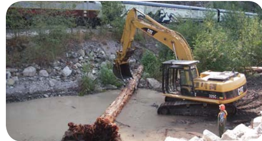
Mile 49 Channel - placement of LWD in an isolated portion
