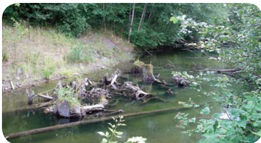
Installed LWD at Paradise Valley Channels
